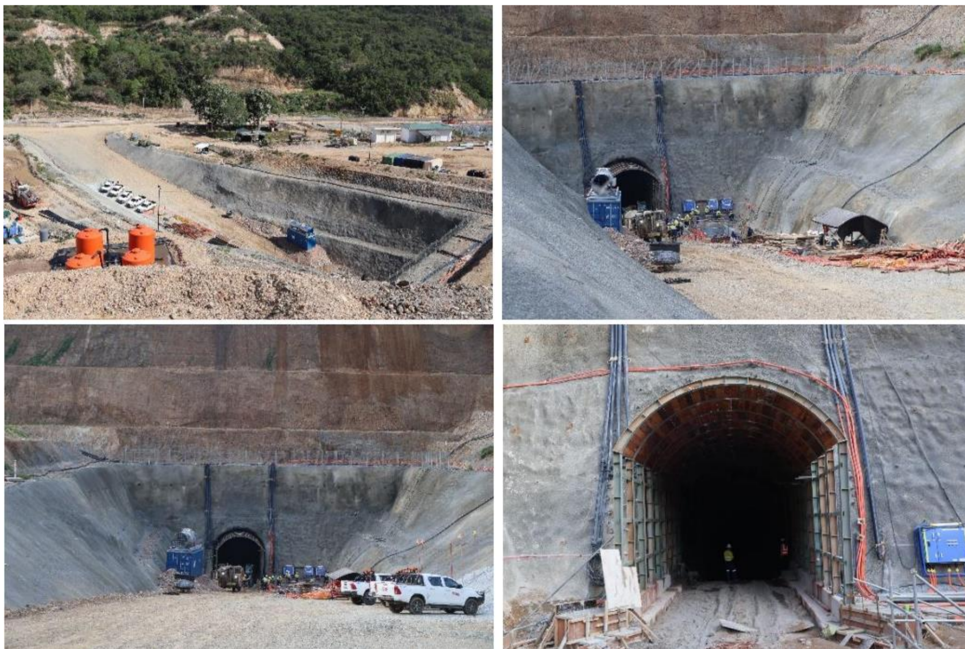
Figure 7. Underground Mining Development
